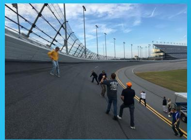
Daytona track has a 31° angle and a possible speed of 170 mph around the turn. The banking of the road allows drivers to take a curve at higher speed.
